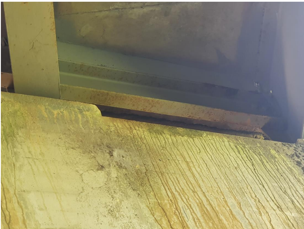
Photo 17: Gaps between concrete slabs on underside of Shadrachs Bridge
