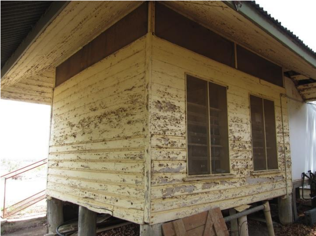
Northeast view of walls and eaves.
