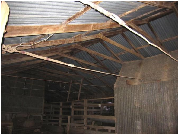
View of interior of roof.
