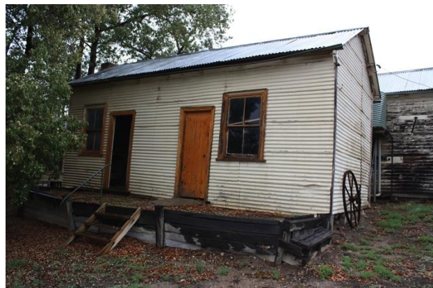
East wall and earth verandah.
