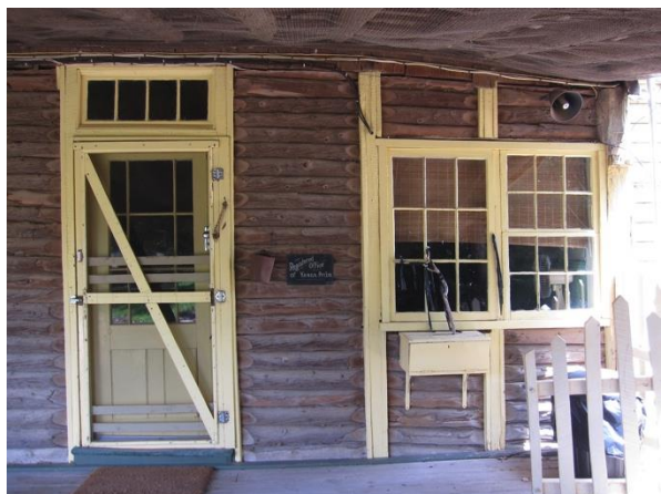
View of north wall of Office with drop log wall panels, door with highlight, windows and Yanga Office sign.
