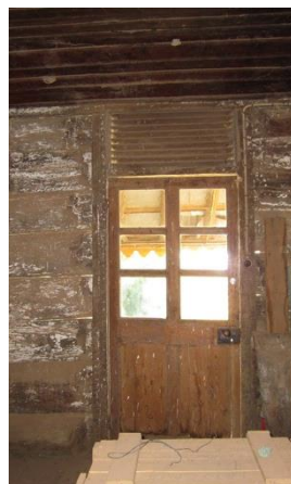
Interior view of Store door and drop slab wall.
