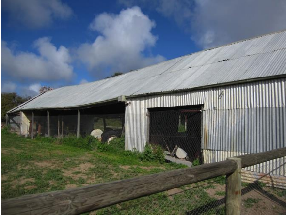
East wall viewed from north.
