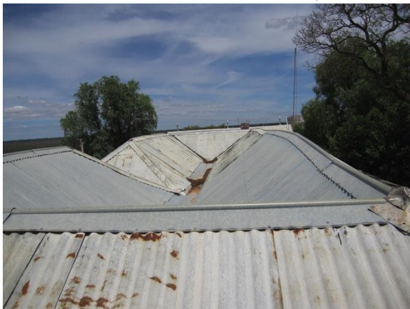
Roof looking west showing central valley.
