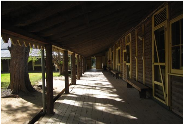
North verandah looking east.
