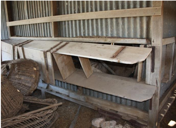
Pigeon holes on north wall of grain store.
