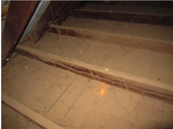
Top of ceiling lining boards from roof space.
