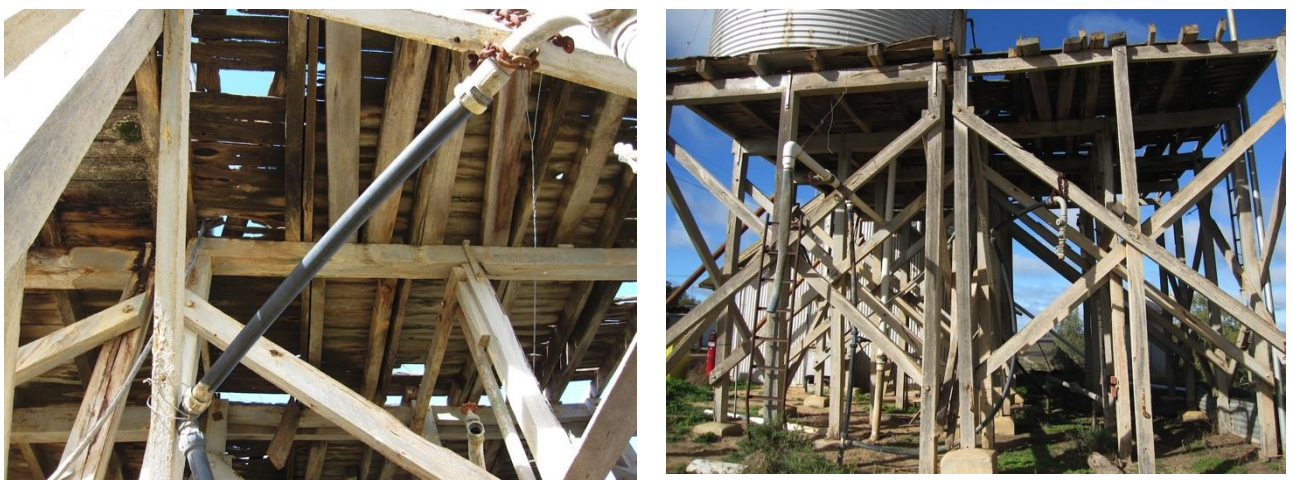
Figure 3.4.31 Views of water tank towers. Photos by CMP authors, 2009
