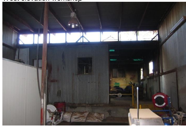
Interior of Machinery Shed.
