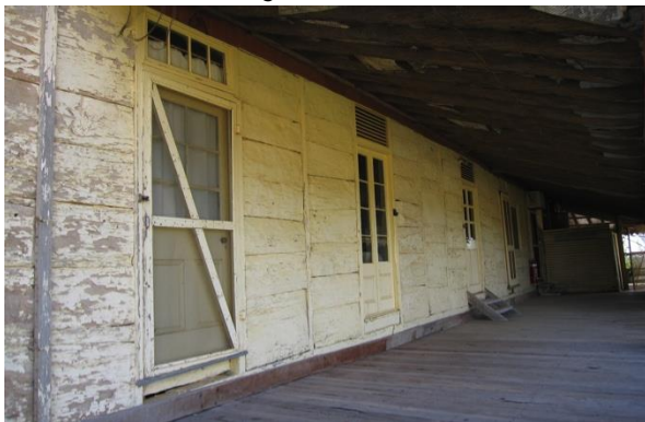
Drop slab wall and south verandah, looking east.
