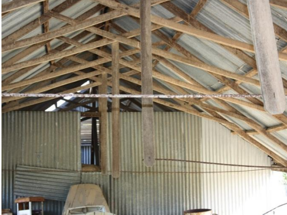
Coach shed interior showing roof structure.
