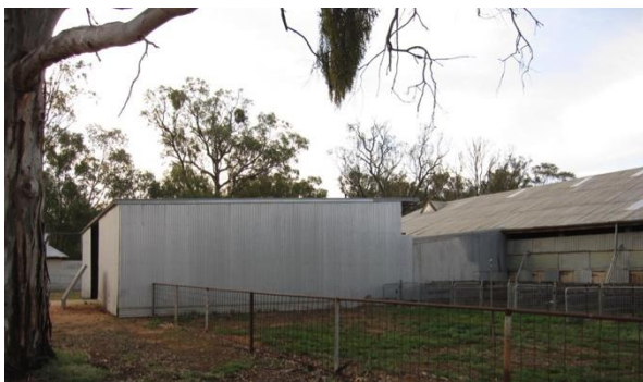
Exterior of Loading Area
