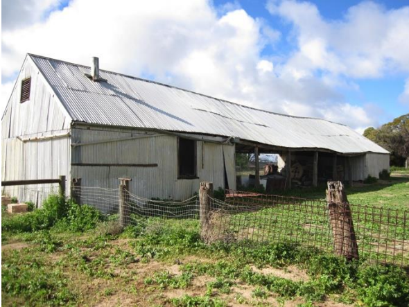
West wall viewed from north.
