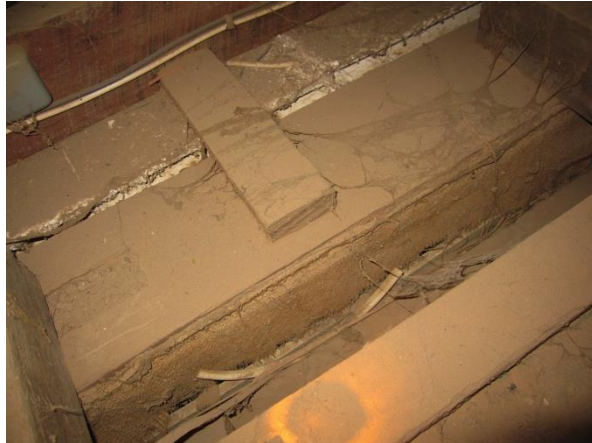
Top plate of wall with remains of hessian wall lining.
