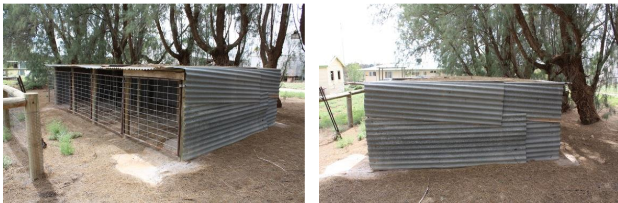
Figure 3.4.49 Views of Kennels. CMP authors, 2009
