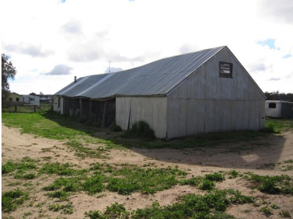
West wall viewed from north.
