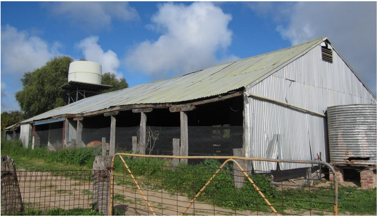
View of east wall from north.
