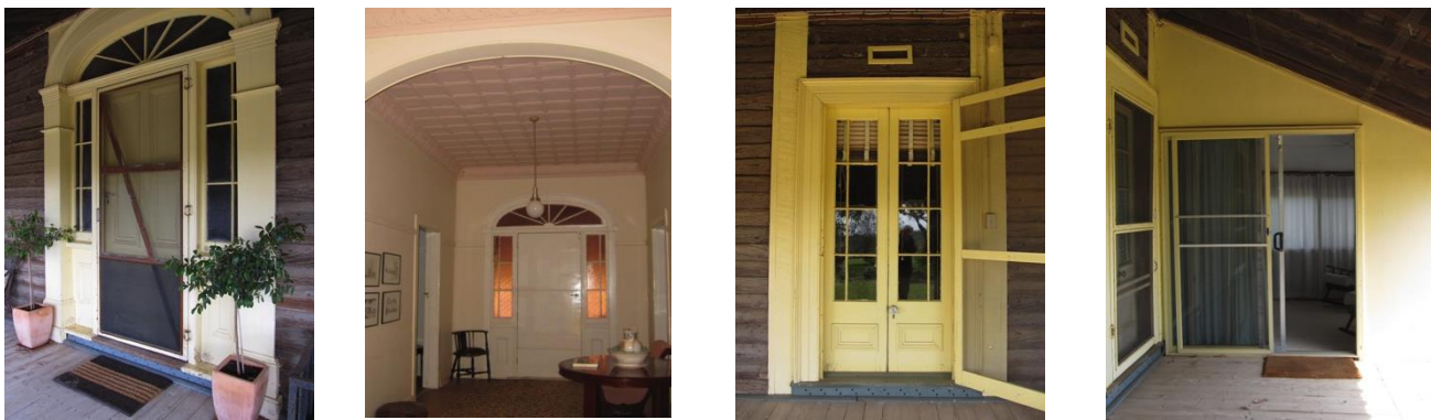
Figure 3.4.6 Front doorset with elliptical fanlight and sidelights - outside and interior views. Typical French door with margin glazing bars and intrusive aluminium door to the Flat. Photos by CMP authors, 2009
