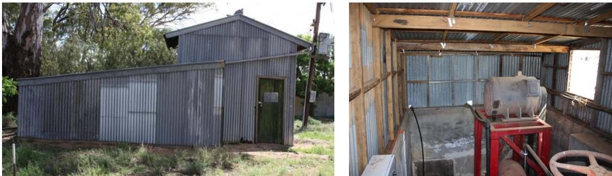
Figure 3.5.26 South west and interior views of Irrigation Pump House. CMP authors, 2009
