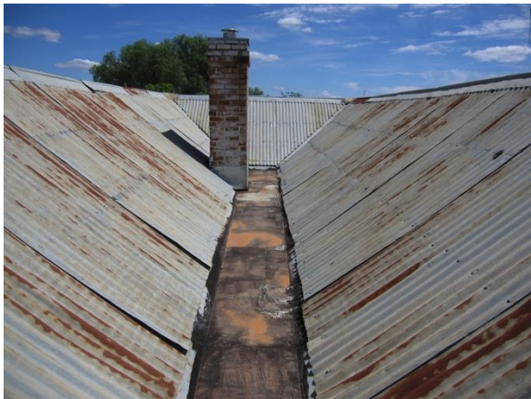
Central roof valley looking north.
