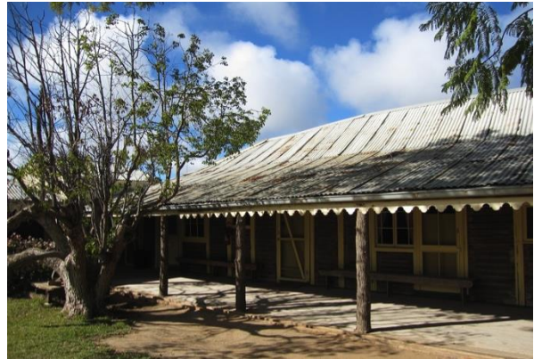
View from north.
