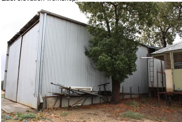
Northeast view of machinery shed.
