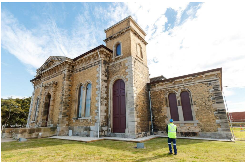
Image: Carrington Pump House post conservation works. Source: Newcastle Herald.
