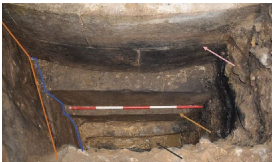
Image: Circular face of the southeast fort tower (pink arrow) above polygonal courses (tan arrow). The c.1820s eastern fort wall (blue line) is below the lowest course of the c.1860s Barbette wall (orange line). Bedrock is at base (black arrow) (note seawater at base). Scale 1m, 200mm increments. (Source: GML Heritage 2023)
