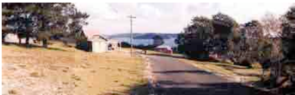
Photo 3.5-8 As the entry road approaches the Administration Precinct, the Pines to the left, remnant Melaleucas to the right and open grass areas denote a transition into the formal landscape of the Quarantine Station.
