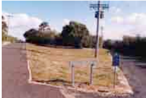
Photo 3.5-5 A lack of formal kerbing characteristics the entry road. The entry takes the right fork, with the exit to left, without destination views.
