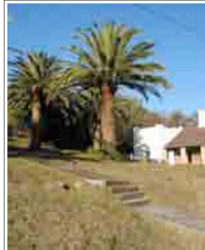
PHOTO 2.2-5 ADMINISTRATION BUILDING A1, 2003 SOURCE: TBLD P/L
