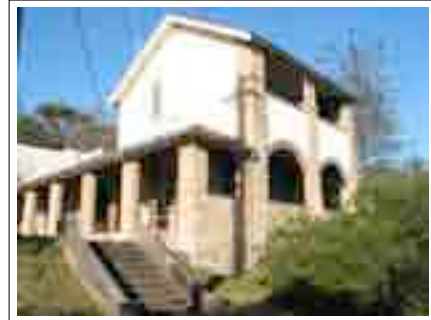
PHOTO 5.5-6 BUILDING A1 TBLD 2003
