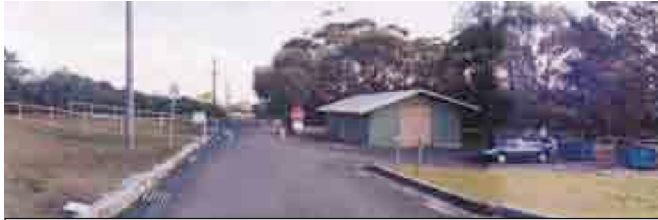
Photo 3.5-1 Entry view to Quarantine Station, characterised by double fences, receiving shed and long straight entry road.
