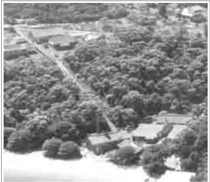
PHOTO 5.1-7 VIEW OF FUNICULAR CIRCA 1940 ILLUSTRATING CLEARED ROUTE OF VARYING WIDTH CIRCA 1940 SOURCE: STATE ARCHIVES
