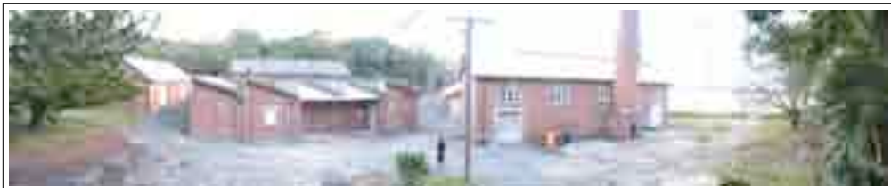
PHOTO 5.1-8 VIEW OF THE WHARF PRECINCT FROM THE PROPOSED LOWER RESTING PLATFORM TBLD 2003
