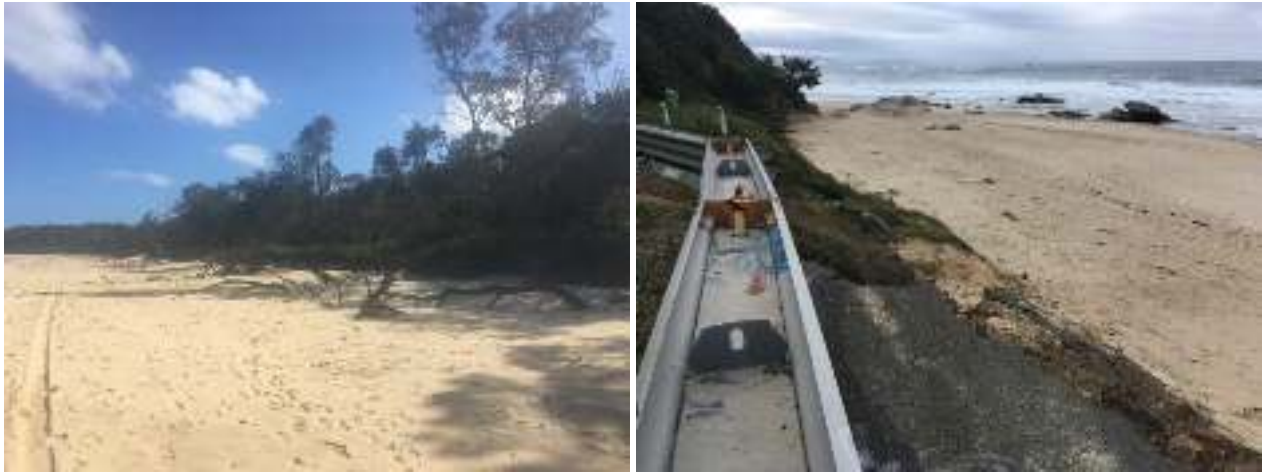
Plate 8: Left: Vegetation debris on receding shoreline north of Swimming Creek entrance (December 2018); Right: recession of beach at Ulrick Drive carpark (north end of Beilby's Beach) causing undercutting and collapse of the road surface (July 2018)
