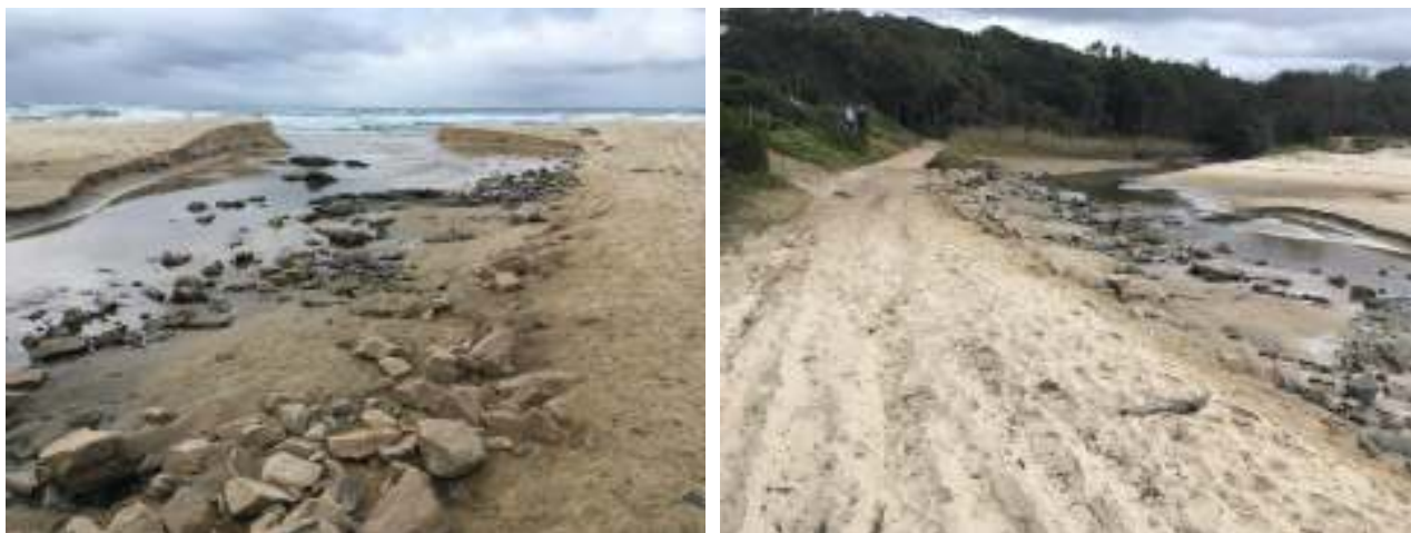
Plate 10: Erosion control at Swimming Creek entrance (September 2018)
