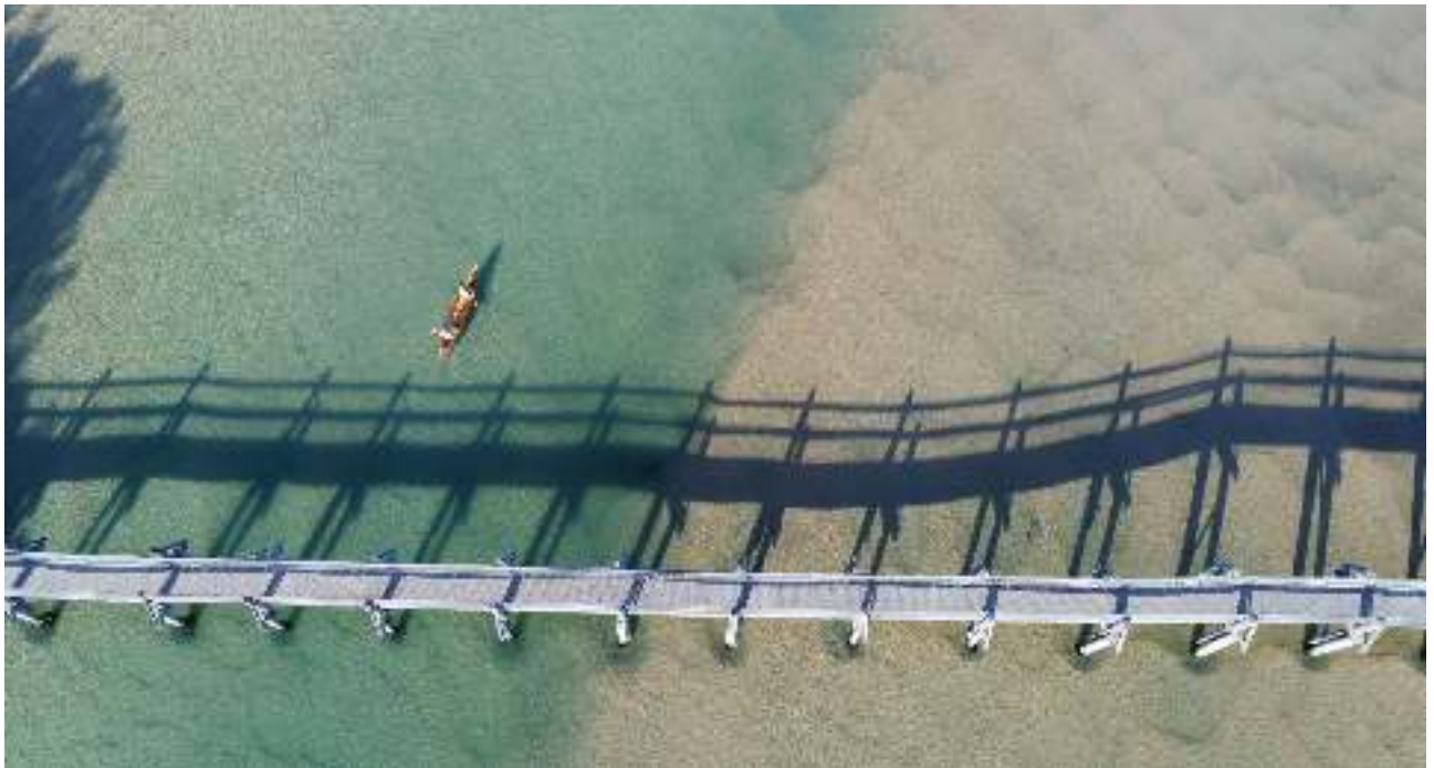
Plate 2: Deep Creek footbridge
