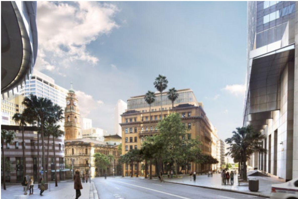
Department of Lands (left) and Education (centre) (Photo credit: Building Review Journal, brj.com.sg )
